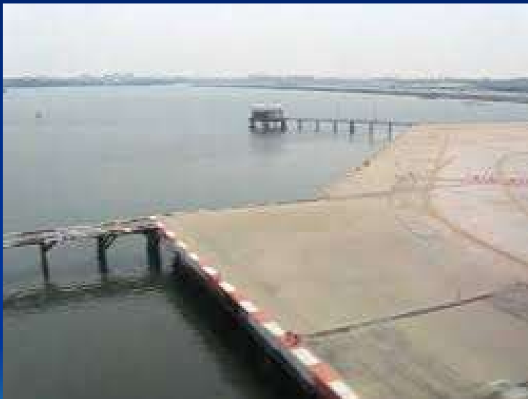
LGA R/W 22 piers
