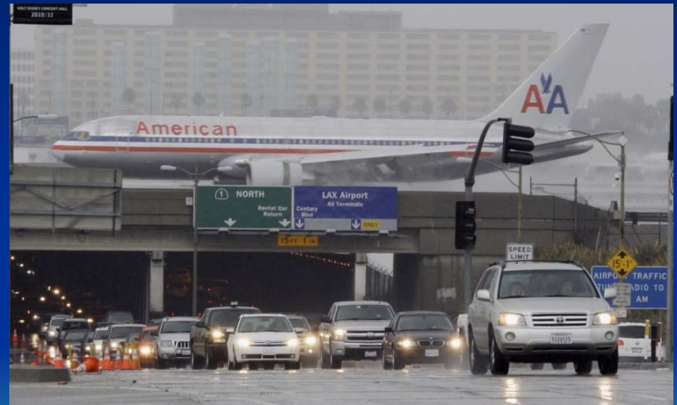
LAX Sepulveda Blvd. tunnel
